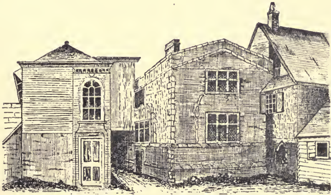
BRIDGE CHAPEL, ROCHESTER (SOUTH-EAST VIEW).
